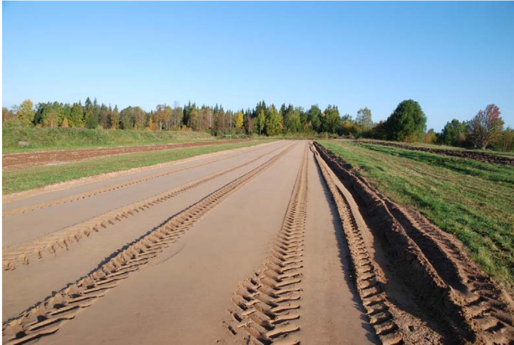
Figure 4: Prepared test lane with the soil compacted. Picture © GICHHD
