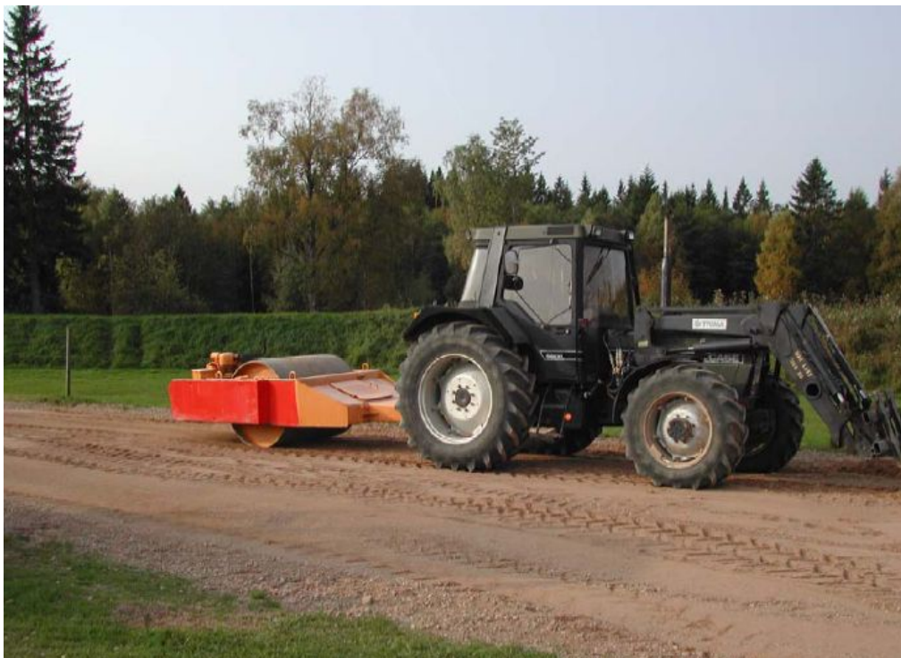
Figure 3: Preparation of standard test lanes – compacting the soil Picture © SWEDEC
